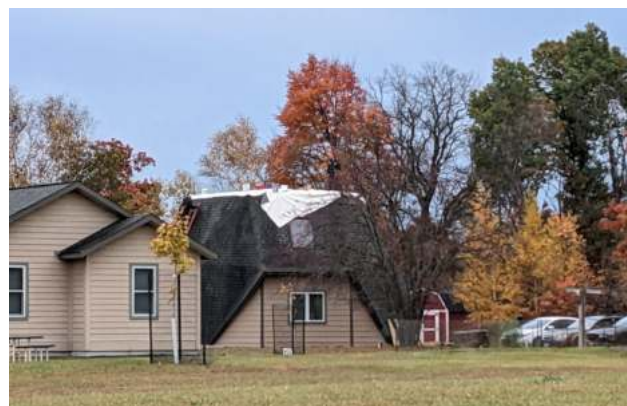
Roof repairs are underway at the Dragonfly Dome House
